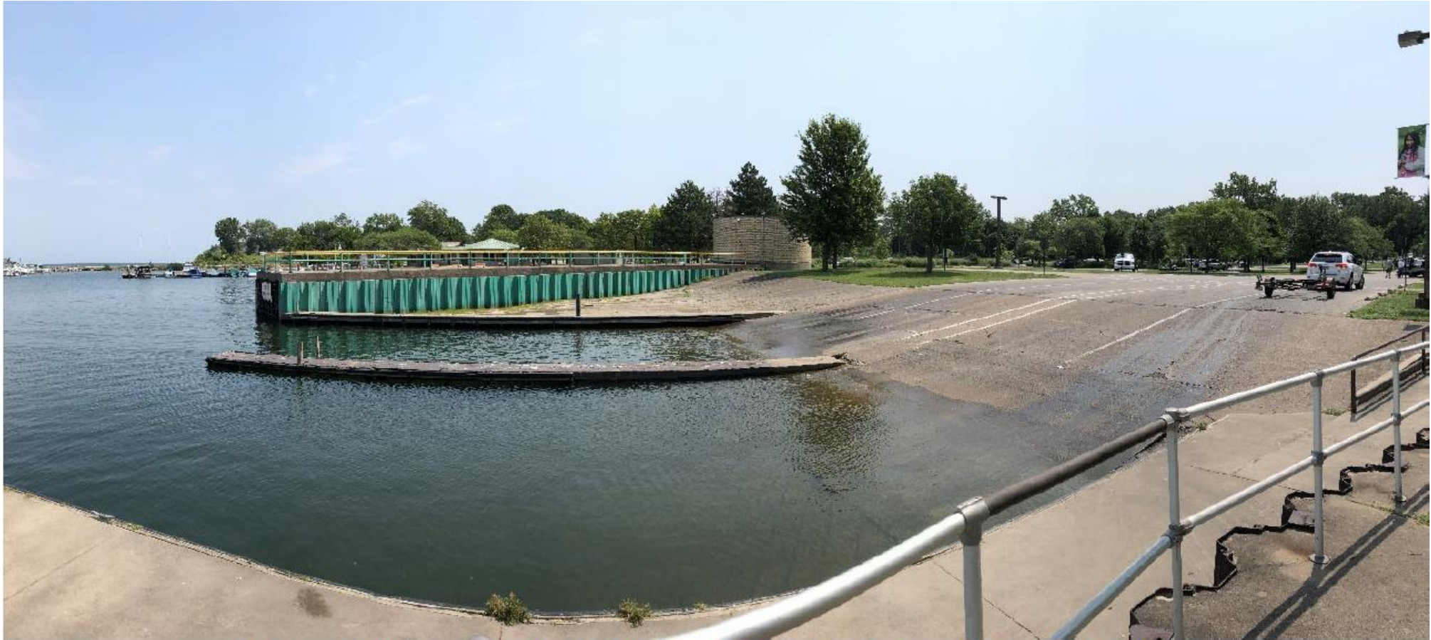
Figure 1: Panoramic View of Wildwood Marina Boat Ramp (KS, July 27, 2021)
