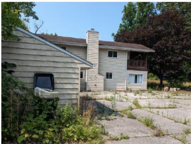
H- Existing house and hardscape to be demolished.
