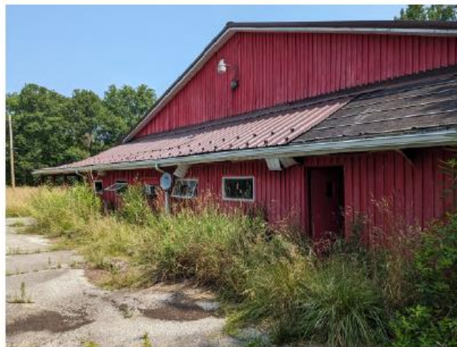
I- Existing barn and hardscape to be demolished.
