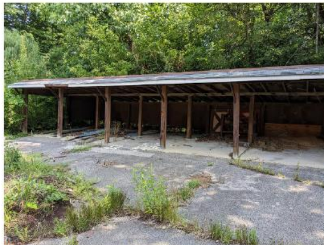
K- Existing house and hardscape to be demolished.
