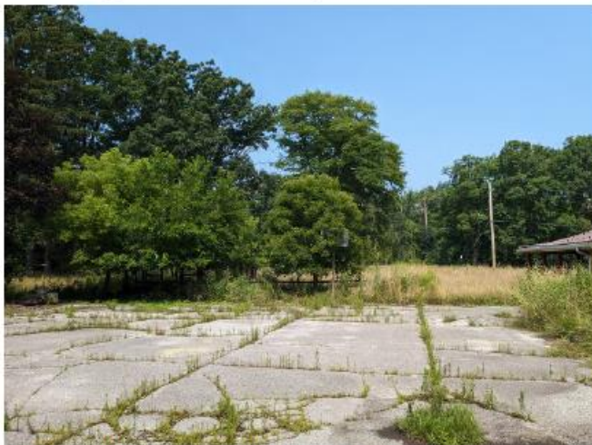
J- Existing hardscape to be demolished.
